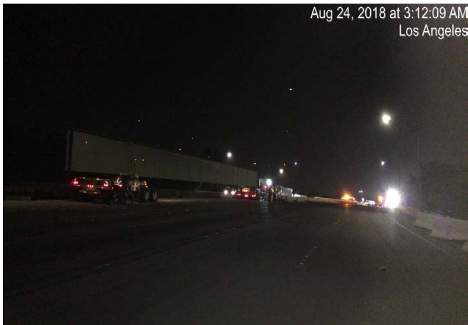
Moving girders to temporary storage area
